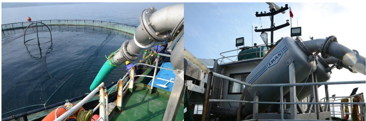
Figure 3. The pipe (left) and pump (right) moves fish in water from the sea cage to the stunner.
